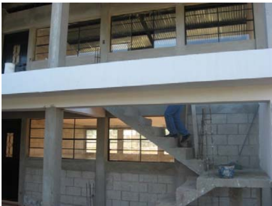
Stairs leading to second story of the 4-classroom school
