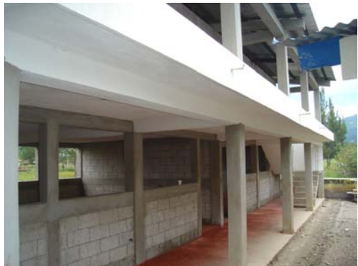
Picture taken before windows and doors were
